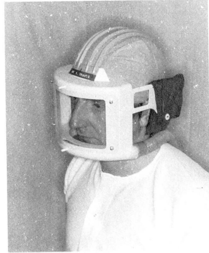
Fig. 11. Headpiece with transparent window and suction hoses.
